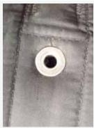
Place grommet through terminal end of housing and cover flap. Set in place. Depending on your grommet setting tool you may need to invert grommet and washer, should that happen the washer spurs need to be flattened prior to setting.
