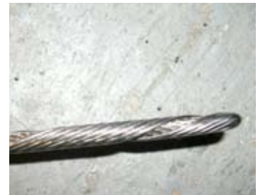
Non-approved metal cable and metal unraveling.
