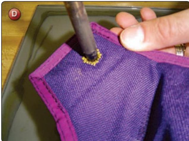
2. Set the grommet in the repaired hole. [Figure E]
